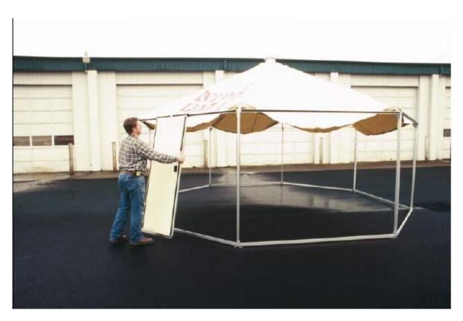
9. Fabric wall panels are marked for their proper placement, "right of door", "left of door", etc. These placements are determined from the outside of the shelter. Starting at either side of the door, apply the wall panels along the eave bars, pulling the panel as tightly as possible along the Velcro strip. Seal the panel to the side of the door. Attach remaining panels by matching colored Velcro ends. Adjust tension of the wall panels by pulling tightly at the wide Velcro section.
