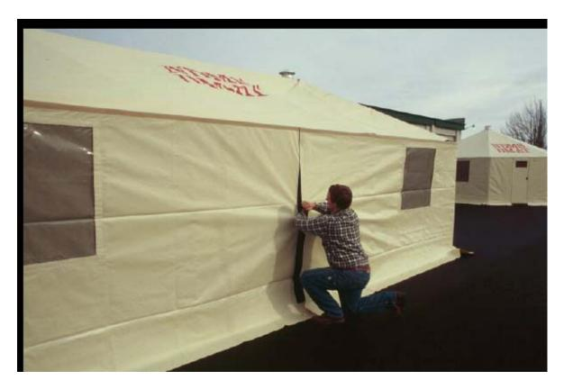
10. Secure roof panel to wall panels with seams lining up with roof trusses. Stretch top as tightly and possible to maximize wind deflection. Stake all leg bars to ground at the leg feet on the inside of the shelter through the stake holes.
