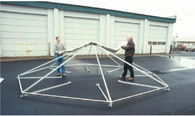
6. With two persons evenly spaced on one side of the frame, gently raise <u>one side</u> of the frame, allowing the leg bars to fold down completely to their vertical position and lock into place with the chained locking pins. Repeat the process with the opposite side of the structure. Position and lock all remaining leg bars.
