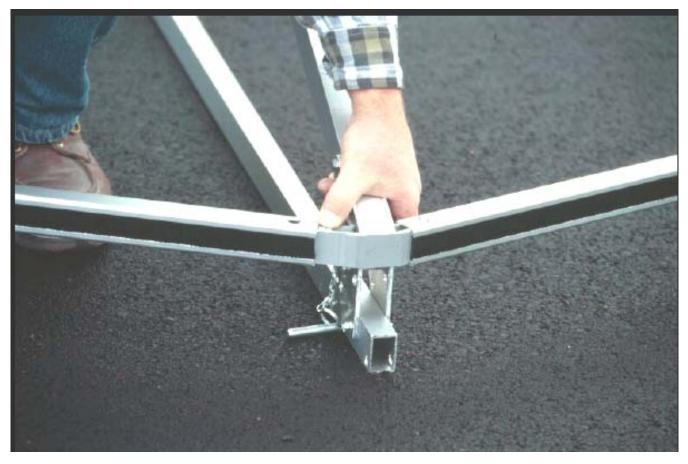
5. <u>Assuring all eave bars are locked into frame</u>, place the roof cover on top of the frame. Unfold the cover to the outside of the frame. Align center of the cone over the center pipe on the top of the frame. Now install the vent cap over the center pipe, pushing down until the cap meets the cone. Hook the 2 springs to the bottom of the key flange. <u>Do not</u> secure the roof to the eave bars at this time.
