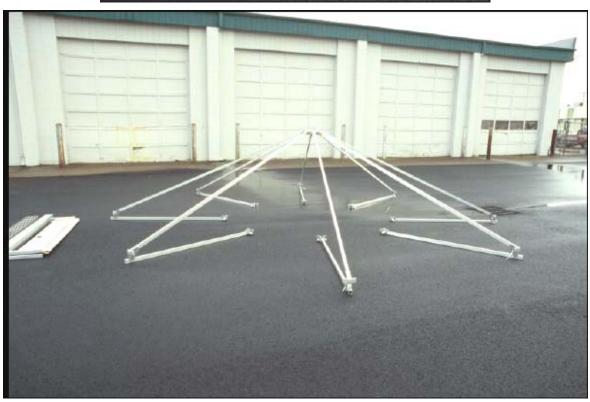
4. Snap in all eave bars with the Velcro side out. If the shelter is on uneven ground, it may be necessary to work them <u>gently</u> in and out and up and down until they lock into position. Never force the fit.
